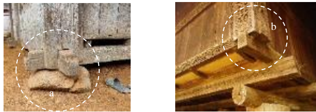
Figure 26. (a) Full two-way neck joint (b) Shallow two-way neck joint
