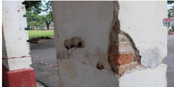
Figure 11: Visual Inspection of the Corridors Area
