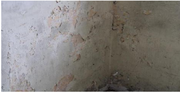
Figure 8: Visual Inspection of the Corridors Area
