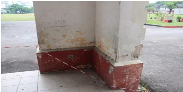
Figure 10: Visual Inspection of the Corridors Area
