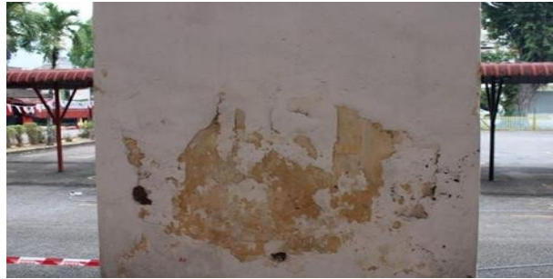
Figure 9: Visual Inspection of the Corridors Area
