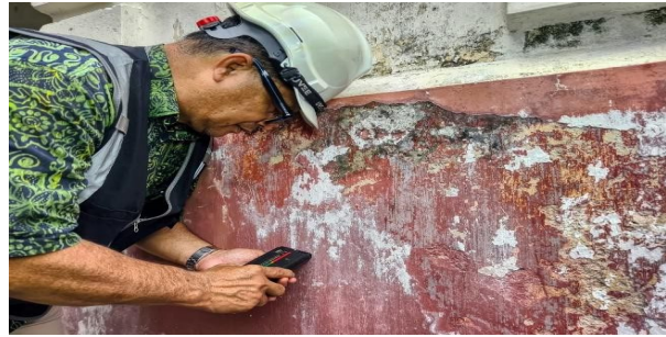
Figure 14: Assist by Conservator to Measure the Moisture
