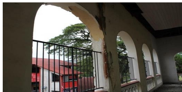
Figure 3: Visual Inspection of the Corridors Area
