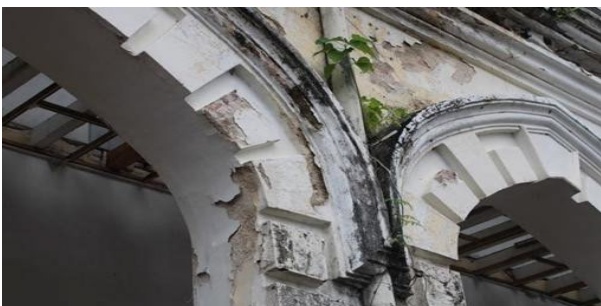
Figure 7: Visual Inspection of the Corridors Area
