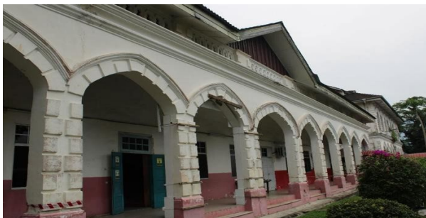
Figure 2: Visual Inspection of the Corridors Area
