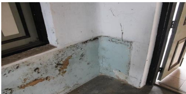
Figure 5: Visual Inspection in the Class Area
