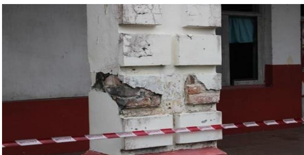
Figure 6: Visual Inspection of the Corridors Area
