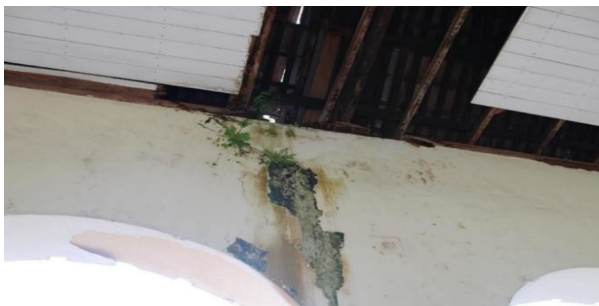
Figure 4: Visual Inspection of the Corridors Area
